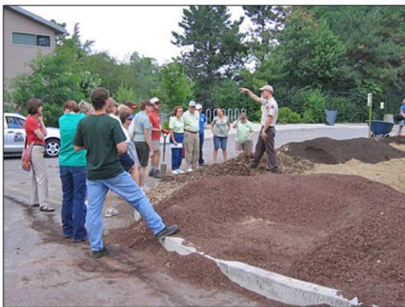
Fig 8. Soil amendments delivered for use in a rain garden Photo by Dave Dyke
