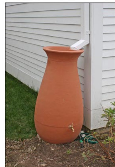
Fig. 5 Rain barrel collecting water from a downspout Photo by Joe Boggs
