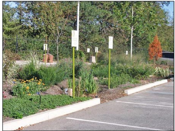
Fig. 3 Curb cut into a rain garden (Photo by Dave Dyke)
