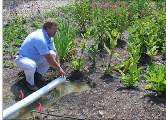
Fig. 4 Rain water piped from downspouts into a rain garden Photo by Joe Boggs
