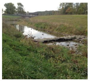
powerful, so put the largest rocks at the base of the stream bank where water velocity is the greatest. Fill voids with various sizes of smaller stone. Do not place filter fabric below the rocks. Plant live stakes (cuttings of willows and other water-loving trees/shrubs) on stream bank slope and trees on top of the slope.
