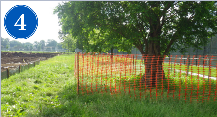
4 Protect trees & sensitive areas with high-visibility exclusion fence.
