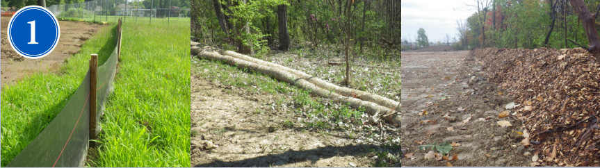
1 Perimeter controls include silt fence, wattles filled with straw or compost, and mulch berms. Check regularly and clean or repair when needed.
