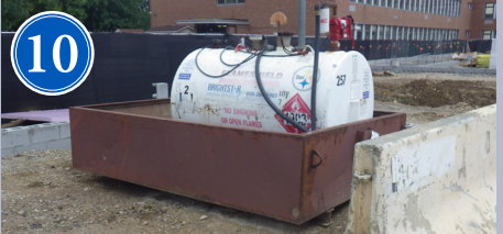
10 Protect fueling areas and know where spill kits and extinguishers are located.
