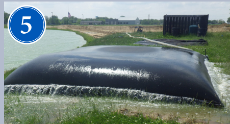
5 Dewatering bags collect sediment from excavation pits
