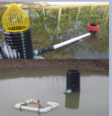
7 Sediment basins are used to collect site runoff to settle out sediments before water is slowly discharged through a surface skimmer. Basins are one of the first practices installed on a site and should be inspected regularly to prevent erosion and ensure outlet structures and skimmers are functioning properly.
