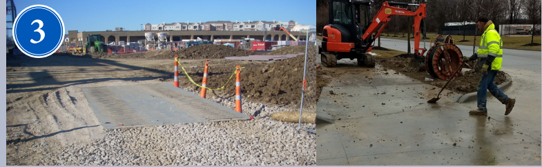
3 Keep entrances clean and safe. Check daily, sweeping up any material.
