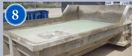
8 Contain concrete, mortar & paint waste.
