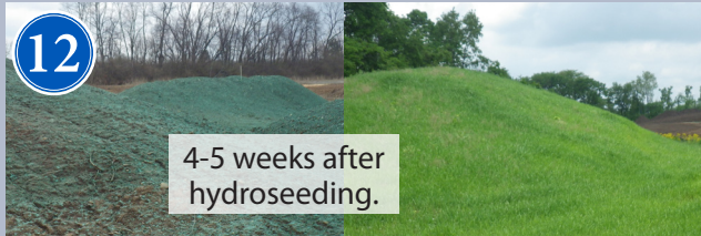
12 Just seed it! Bare soil should be stabilized as soon as possible with seed, straw, blankets or sod to prevent erosion.
