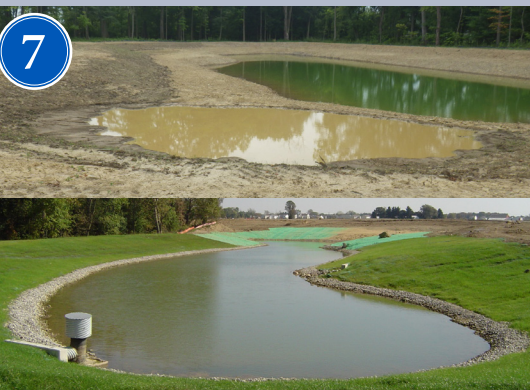
7 Sediment basins are used to collect site runoff to settle out sediments before water is slowly discharged through a surface skimmer. Basins are one of the first practices installed on a site and should be inspected regularly to prevent erosion and ensure outlet structures and skimmers are functioning properly.
